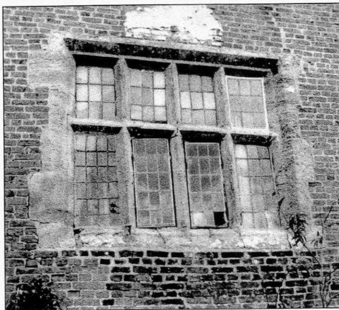
PLATE 33 (above, left): Four-light transomed window of first chamber on first floor of service wing. PLATE 34 (above, right): Tall, unusual cross window of early 1700s on rear wall of wing lights both kitchen and cheese room
