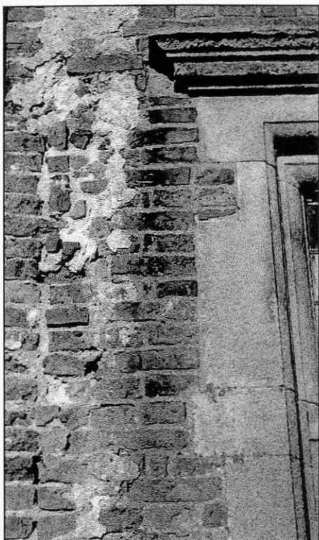
PLATE 19 (left): Rebuilding on corner of west wing indicates where side wall of upper wing was removed
