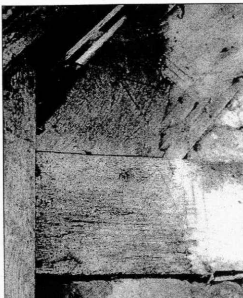
PLATE 101 (left): Carpenters marks VIII on principal rafter and tiebeam of same building
