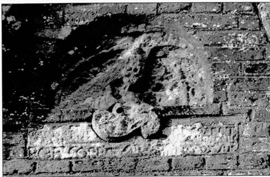
PLATE 16 (above): Attractive dentilation on gable of west wing. Contrast between brick and stone produced the 'red and white' effect popular in gentry mansions at that time
