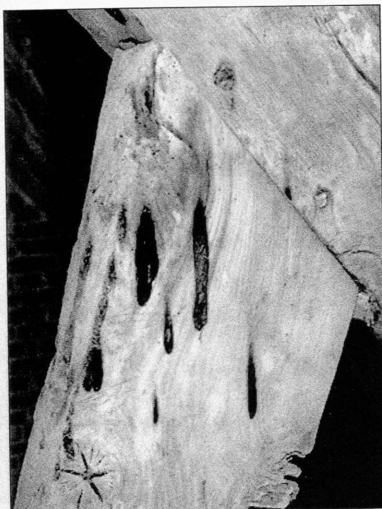
PLATE 91 (above): Stub remaining in principal rafter mortice indicates purlin was removed to allow access to bell tower – proving latter is an addition. Also, brick flue from fireplace in breakfast room and chamber above, unusually angled to join flue of kitchen hearth – shows this too was probably added later
