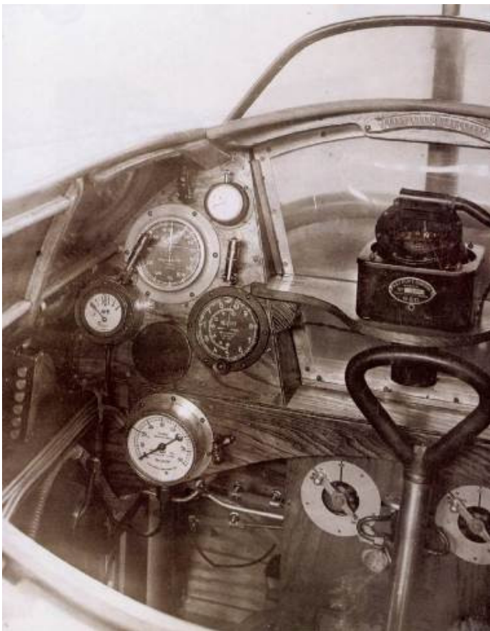
Cockpit of the FE2d showing the characteristic spade grip of the control column, the altimeter, air speed indicator, air pressure gauge and a watch.
